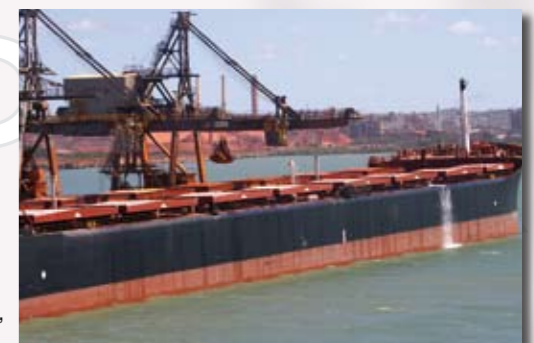
Port loading terminal, Gladstone QLD.
